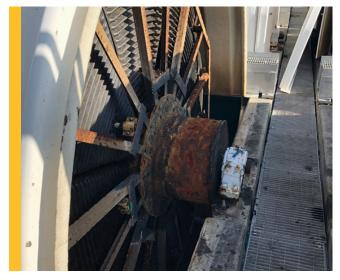
Because RBCs operate so slowly, equipment failure often isn't found until it's too late. The failure on this RBC wasn't found until the media assembly shifted, contacting the concrete and tripping the motor.
