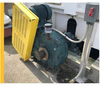
In addition to switching to Safety Mount for its superior seals and quick installation, the plant transitioned to a complete Dodge drive package with BioDisc gear reducers and desiccant breathers for enhanced reliability and valuable savings.
