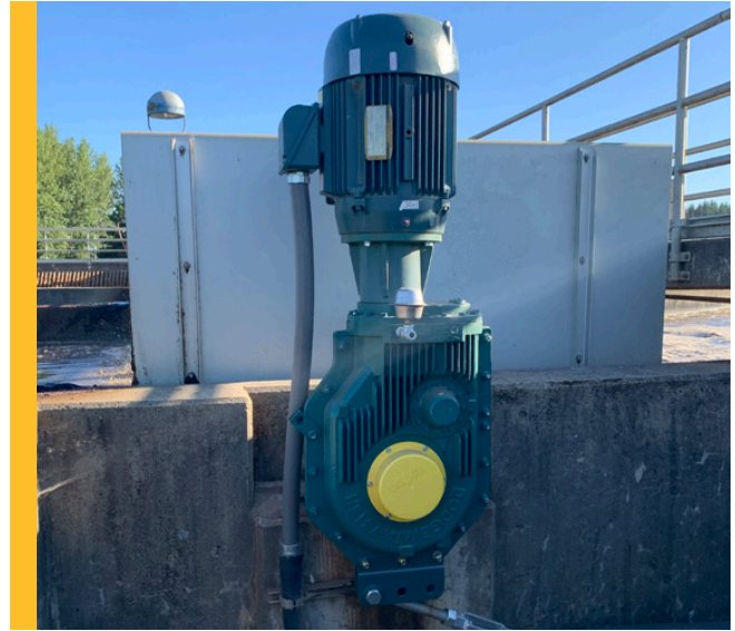
MTA replaced the competitive gear reducer to convert the application to a direct-drive system, providing improved reliability and easier maintenance.
